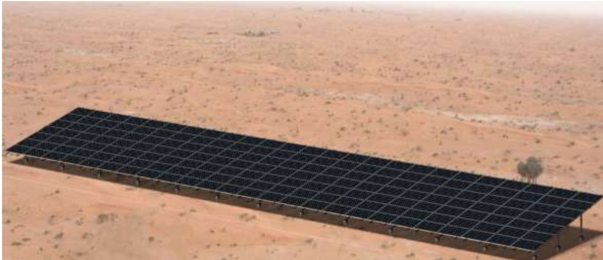
Typical 25 kW Array Installation
